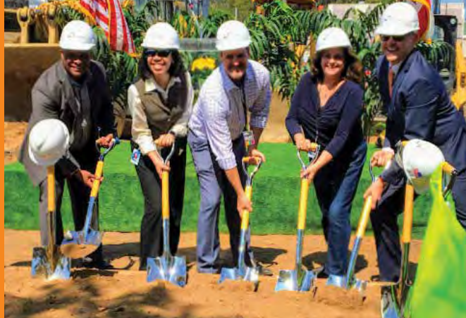
BREAKING GROUND Dr. Eure, Ms. Woo, Mr. Richardson, and Ms. Blanchard participate in the ground breaking as they dig the foundation for the new auditorium. Photo: Clemente Ortiz
