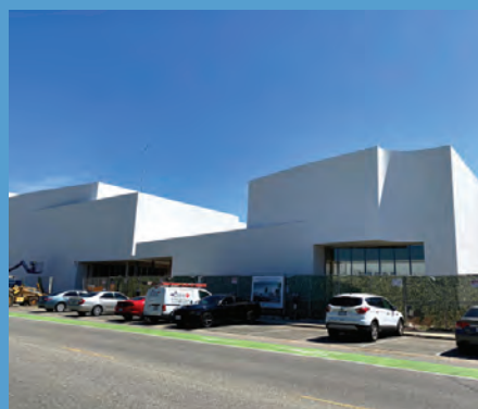
The new complex in progress.
